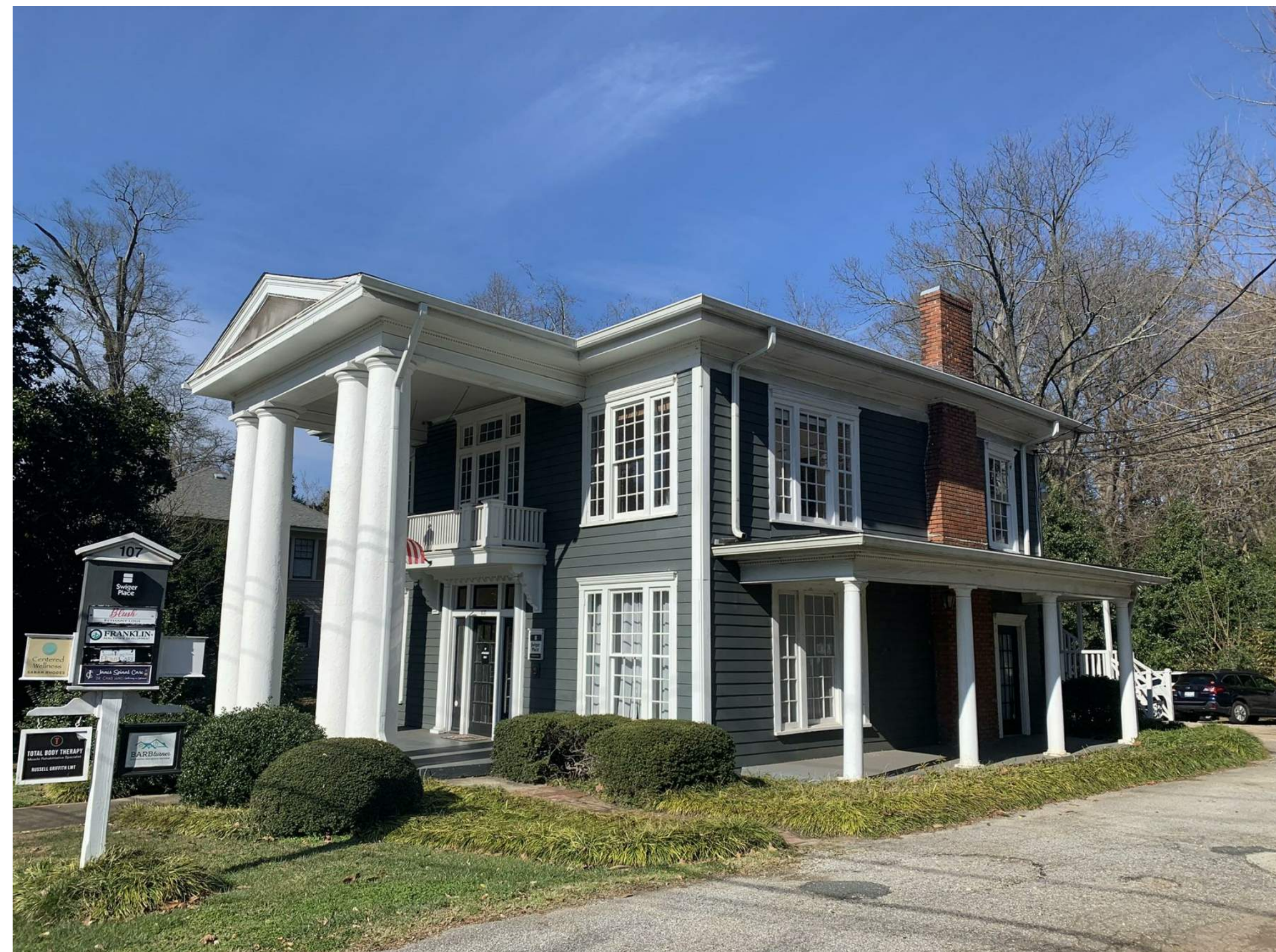
EXISTING VIEW FROM SIDEWALK
